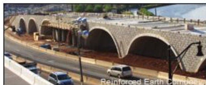
Components of the arches required separate forms and attention to detail.
